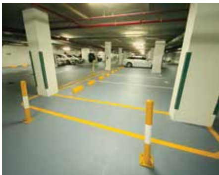
FLOOR EPOXY COATING & ROAD MARKING OF G+7 BUILDING A-B-C
