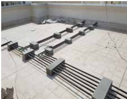
REPLACEMENT OF G+4 BUILDING DOMESTIC WATER SUPPLY LINE
