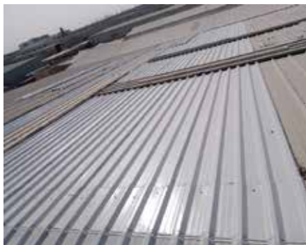
REPLACEMENT OF DAMAGED ROOFING PANELS FOR WAREHOUSE
