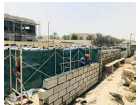
CONSTRUCTION OF BLOCK WALL FOR LE MERIDIEN HOTEL GARHOUD DUBAI
