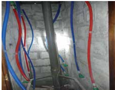
REFURBISHMENT OF G+7 BUILDING DOMESTIC WATER SUPPLY LINE
