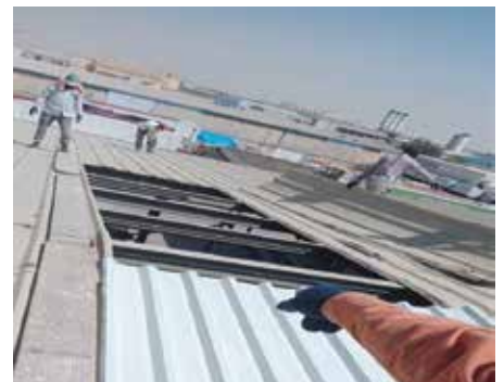
REPLACEMENT OF DAMAGED ROOFING PANELS FOR WAREHOUSE
