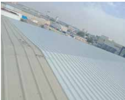
REPLACEMENT OF DAMAGED ROOFING PANELS FOR WAREHOUSE
