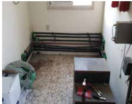
REPLACEMENT OF G+4 BUILDING DOMESTIC WATER SUPPLY LINE
